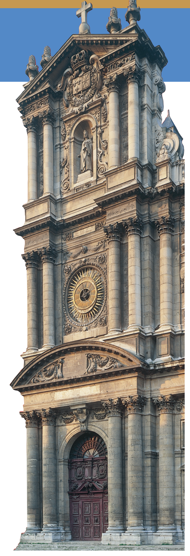
Figure 14 ▲ Detail of the facade of the Church of Saint-Paul et Saint-Louis, Paris. Although not built by the Jesuit Martellange, the three-story facade divided into three sections recall a 1625 project by Martellange, which also had three stories of superimposed columns and a narrow upper section crowned by a cornice.
