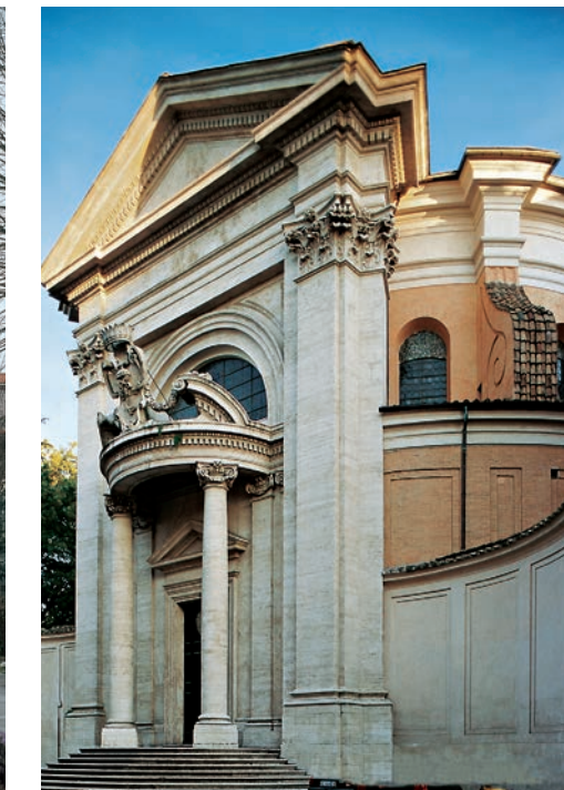
Figure 13 ▲ Exterior of the Church of Sant’Andrea al Quirinale. Bernini’s masterpiece is the Jesuit novitiate church in Rome (1658–70).
